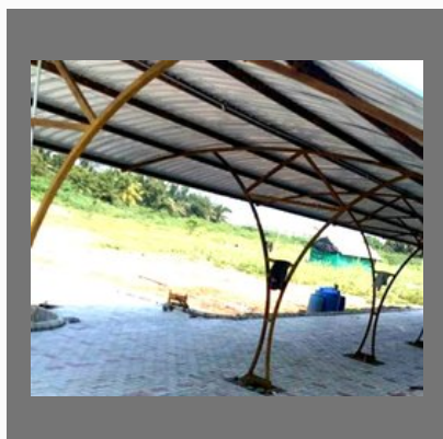
Arch type car parking shed
