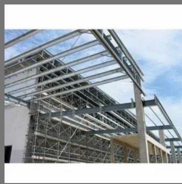
Building Structure Fabrication Work
