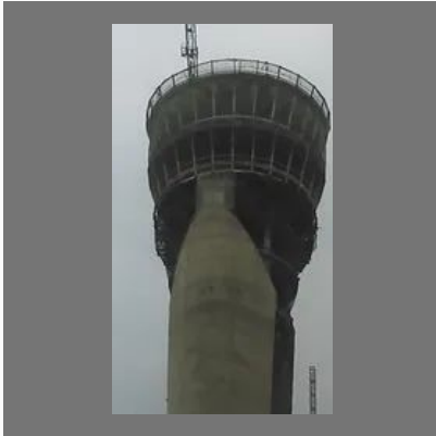
Steel Structure Lift
