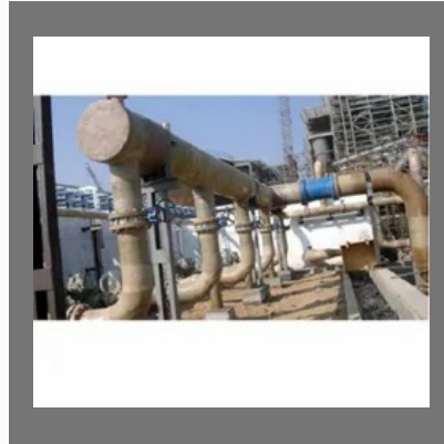
Pipeline Work Services
