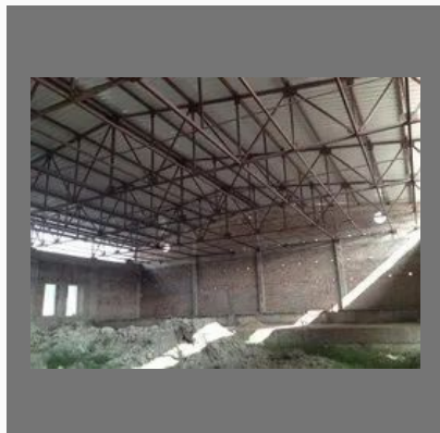
Truss Work Service
