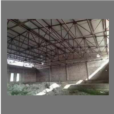
Roofing Sheet Fabrication
