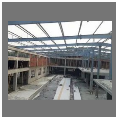
Prefabricated Factory Shed
