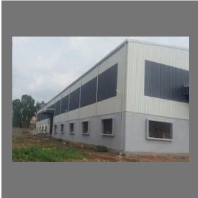
Commercial Complex Construction
