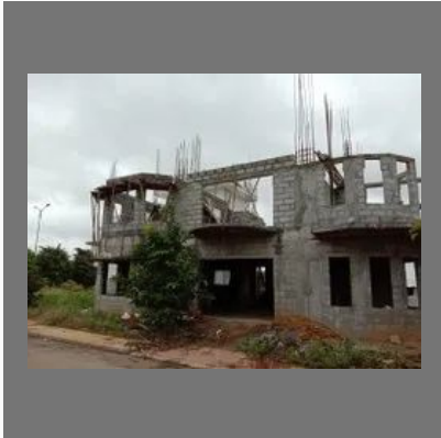
Building Construction Work
