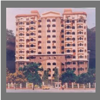
Opg Chs Residential Building Construction
