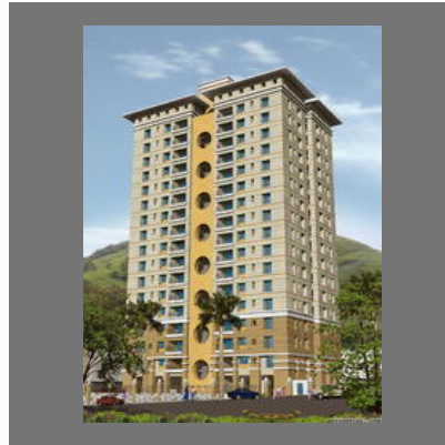
Faculty Housing Building Construction
