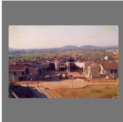
District Court Building Construction
