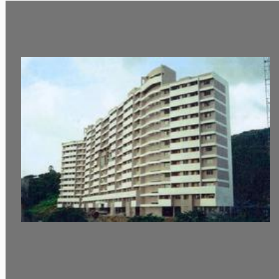
Efficiency Apartments Construction
