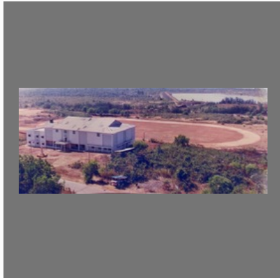
Sports Complex Construction
