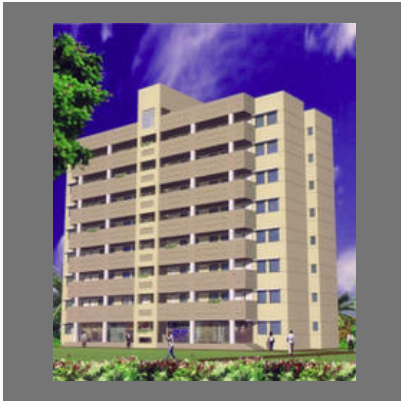
Slum Rehabilitation Buildings Construction
