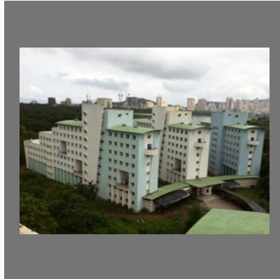
Hostel Building Construction
