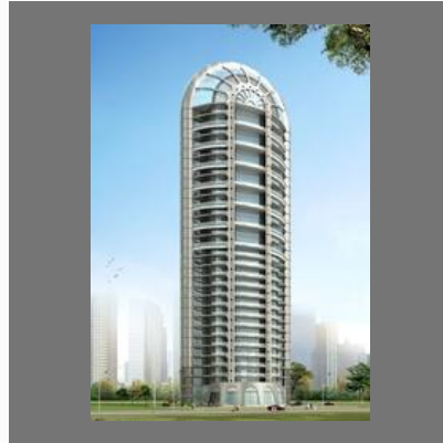
Residential Building Construction
