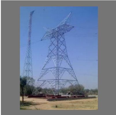
Tower Testing & R D Center
