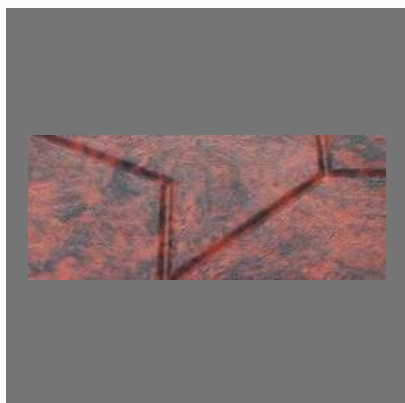
Concrete Sidewalk Slab
