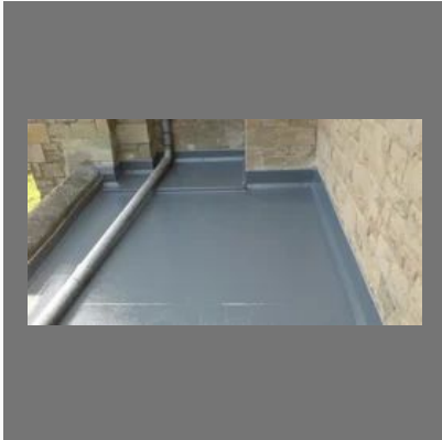
Liquid Applied Membrane Waterproofing Service
