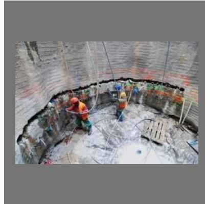
Pressure Grouting service
