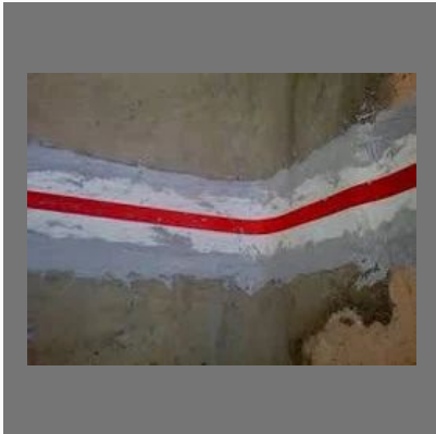
Expansion Joint Treatment
