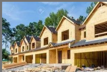
Rowhouse Construction Work
