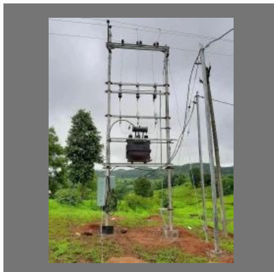
Transformer Installation Service
