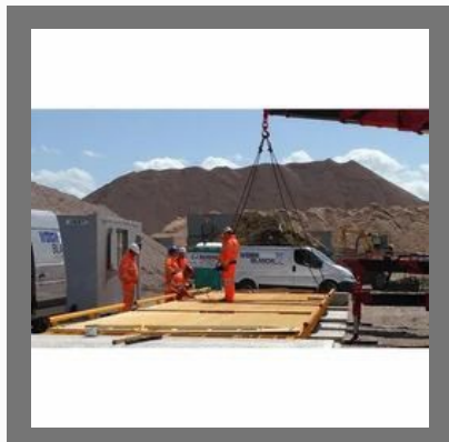
Weighbridge Repairing Service
