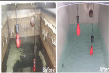
Water Tank Cleaning
