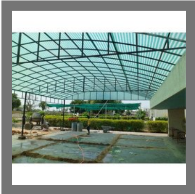
FRP Industrial Roofing Shed
