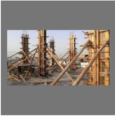
RCC Construction Without Material
