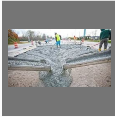
Concrete Road Construction
