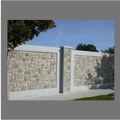
Wall Compound Construction Service
