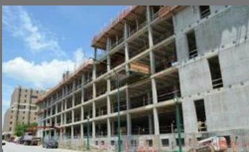
School Building Construction
