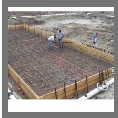
Sewage Treatment Plant STP
