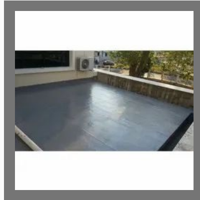
FRP Lining and Coating
