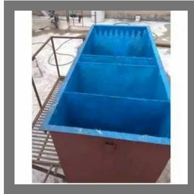
ETP Tank FRP Lining & Work
