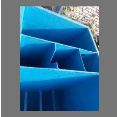
Tank FRP Lining Services
