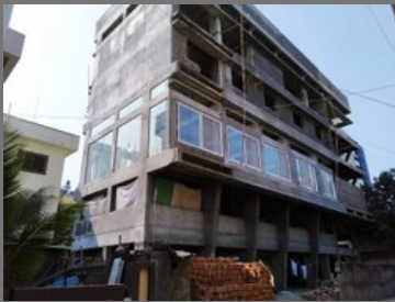
Infrastructure Construction Services
