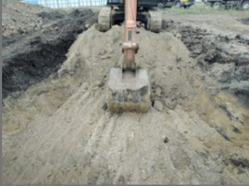
Bridge Construction Service
