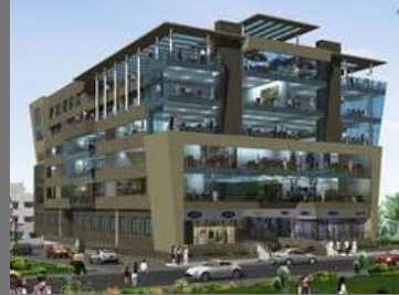
Commercial Complex Construction
