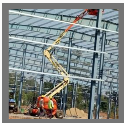
PEB Structural Shed
