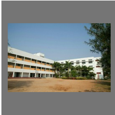
School Building Construction Service
