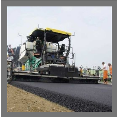
Asphalt Road Construction Services
