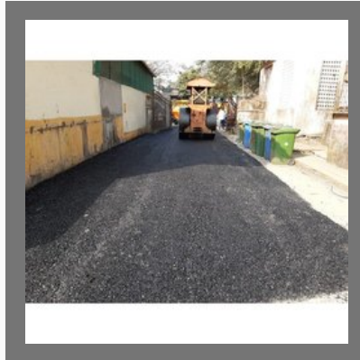
Road Construction Services
