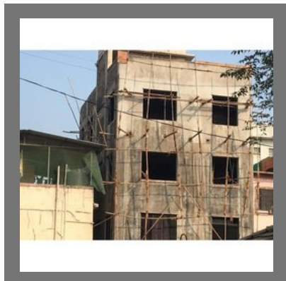
Commercial Buildings Construction
