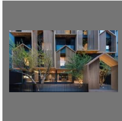
Apartment Interior Designing Services
