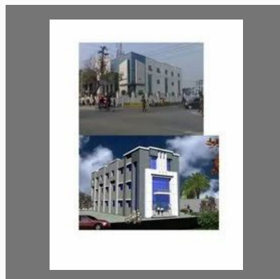
Construction Of Commercial Building
