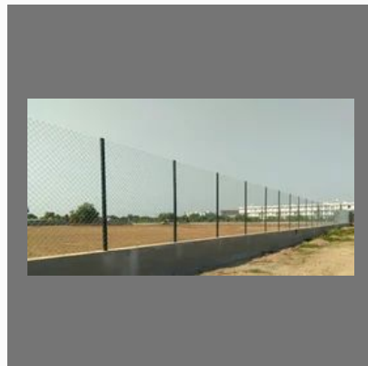
Chain Link Fencia
