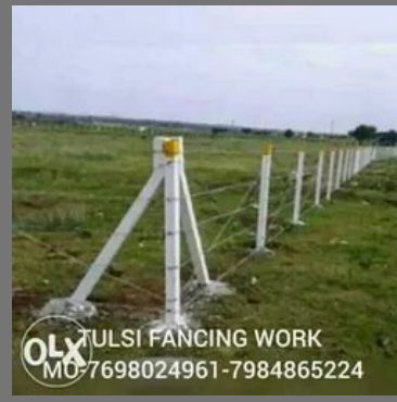
Barbed wire fencing
