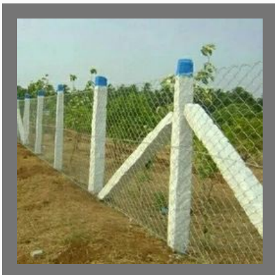
Chain link fencia
