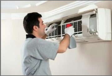
Air Conditioner Repairing Service
