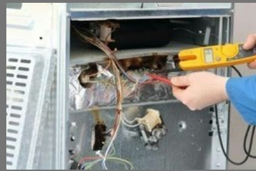
Cooler Repairing Service
