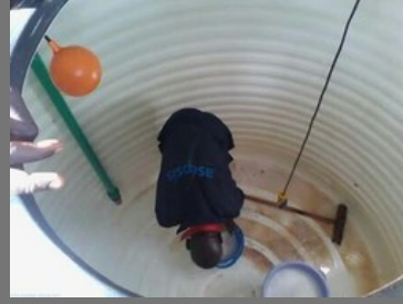
Water Tank Cleaning Service
