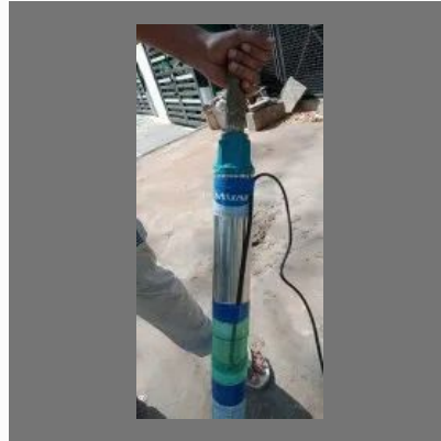
Submersible Pump Repairing
