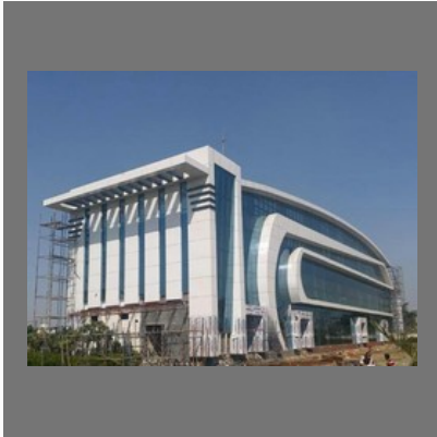
Exterior Wall Cladding
