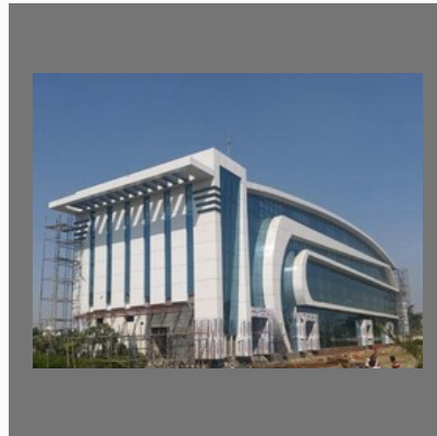
Exterior Wall Cladding
