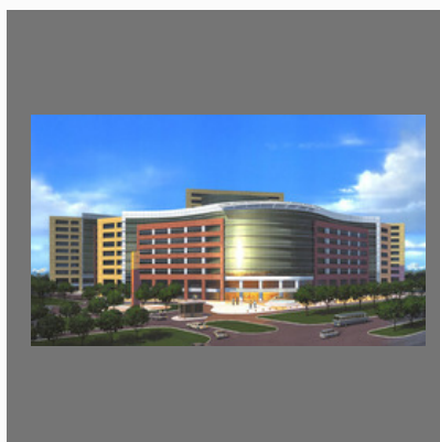
Commercial Tech World Construction in Gurgaon
