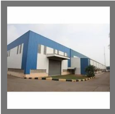
MS Steel Prefabricated Structure
