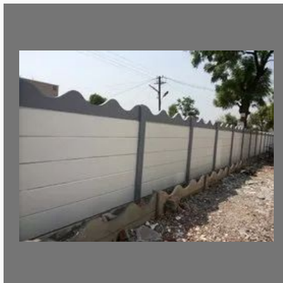
Precast Compound & Fencing Wall
