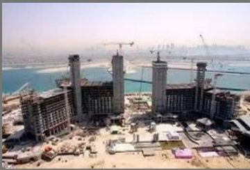
Hotel Construction Service
