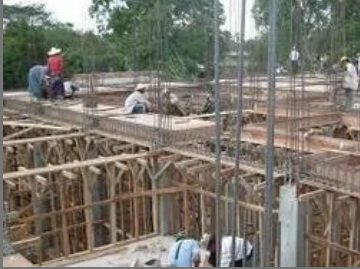
Hospital Construction Service
