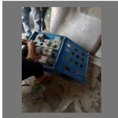
Control Panel Repair Services
