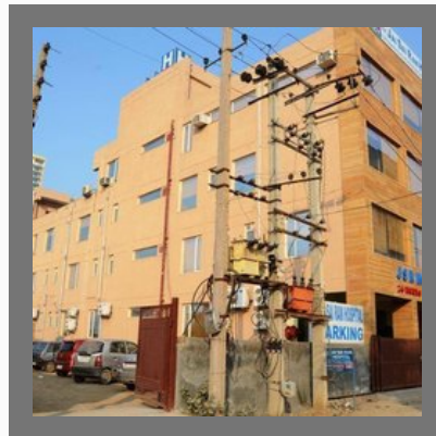
Hospital Build and Design Turnkey
