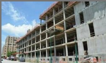
School Building Construction
