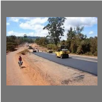
Construction of Roads
