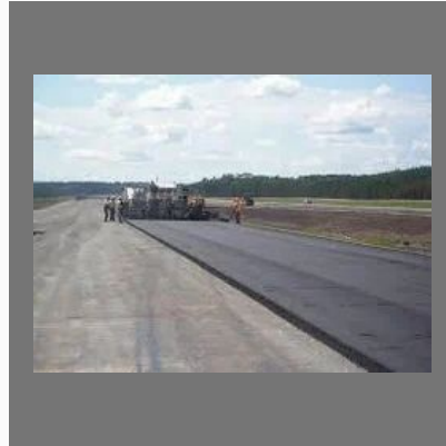
Construction of Highways
