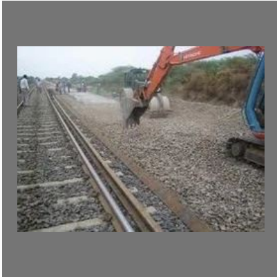
Railway Work Of Kadappa - Bangalore Line
