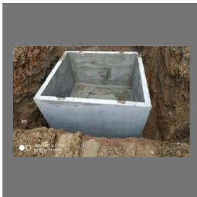
RCC Underground Sump
