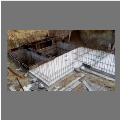
STP Construction Services
