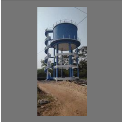
RCC Over Head Tanks
