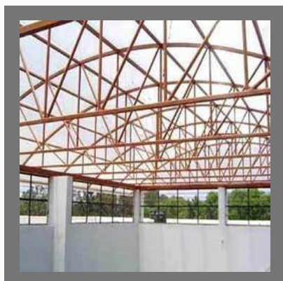
Mild Steel (MS) Fabrication
