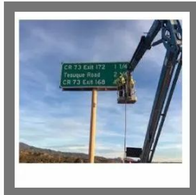
Overhead Gantry & Cantilever Sign
