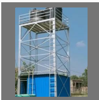
Water Storage Tank Heavy Structural Stand
