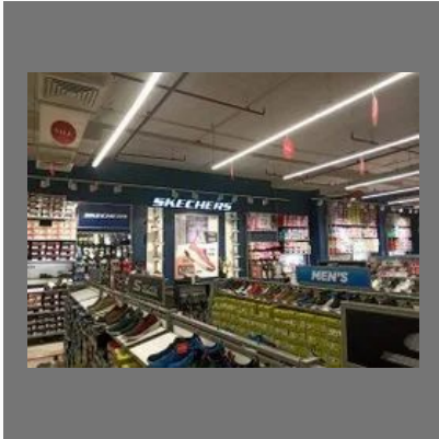
Light Wiring Work
