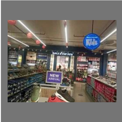
Light Wiring Work
