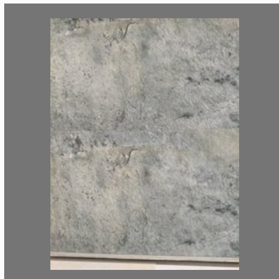
Bathroom Plain Tiles
