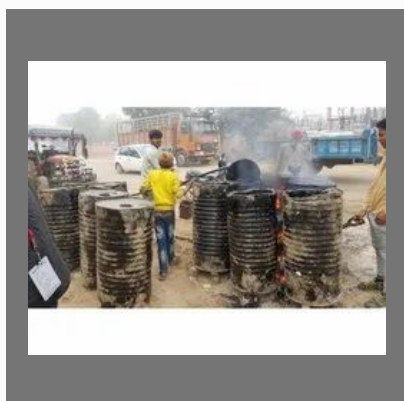
Bitumen Road Construction Services
