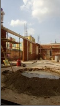
Civil Construction Contractors
