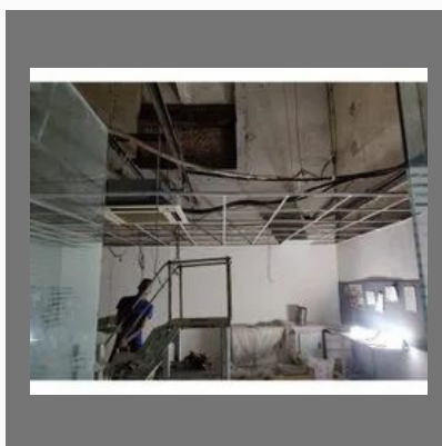
POP False Ceiling Service
