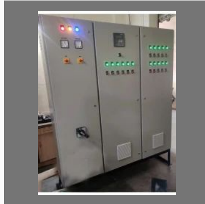
MCC Electrical Control Panel
