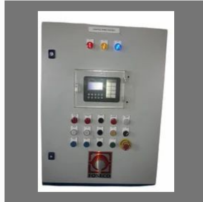
Control Panel Installation Service
