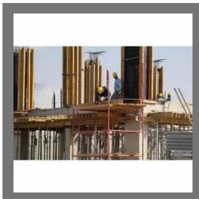
Industrial Building Construction Services
