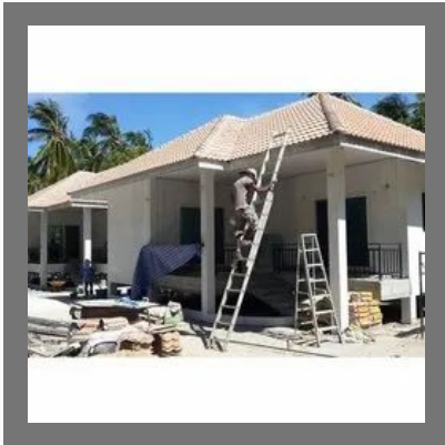
Bungalow Construction Service
