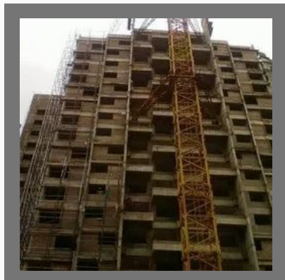
Commercial Buildings Construction
