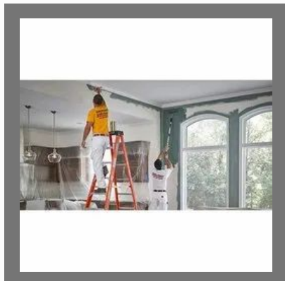
Interior And Exterior Painting Service
