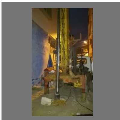
Motor Lifting Erection Job Work
