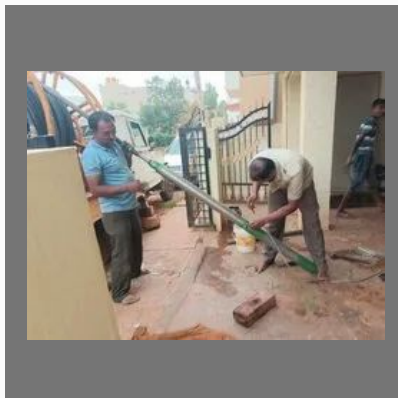
Submersible Pump Repairing Service
