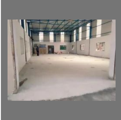
Factory Shed Construction Service
