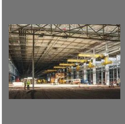
Industrial Project Construction Service
