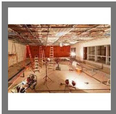
Industrial Electrical Project Work
