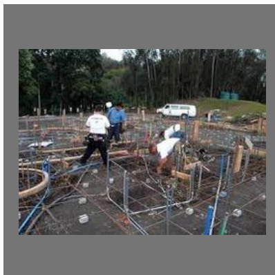
Domestic Electrical Project Work
