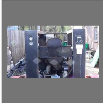
Refrigerated Air Dryer Repair Service
