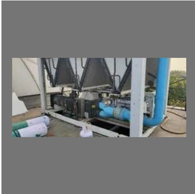
Chiller Plant Repairing
