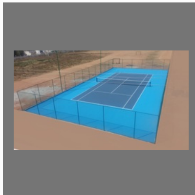
Tennis Court Construction
