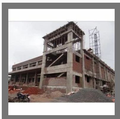
Commercial Building Construction
