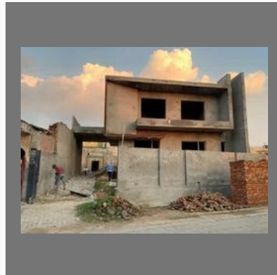
Warehouse Construction Services
