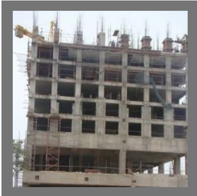
Hotel Construction Service
