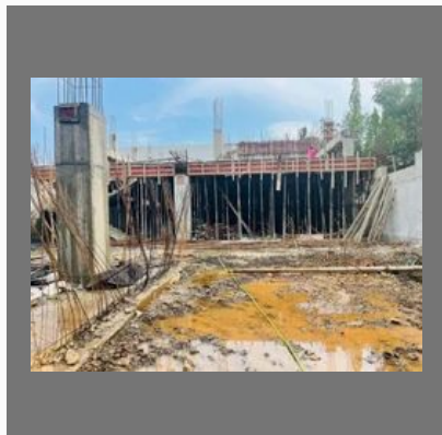
Commercial Construction Service
