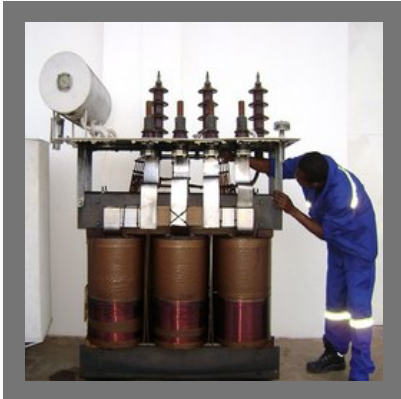
Transformer Repairing Services
