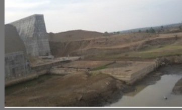
Kal River Dam Construction
