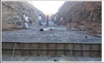
Jamda Dam Project
