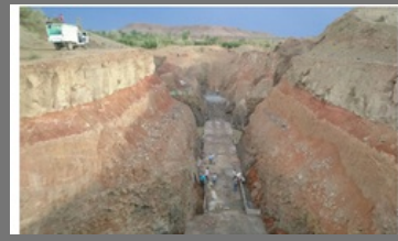
Balganga River Dam Project
