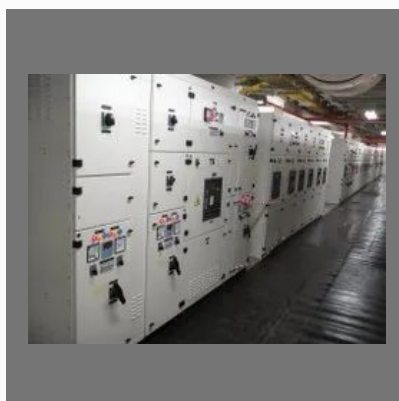
Electrical Structural Work
