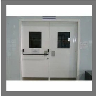
Hospital Operation Theater Door
