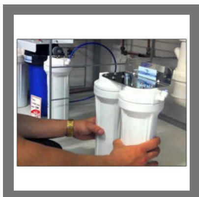
RO Water Purifier Installation Service
